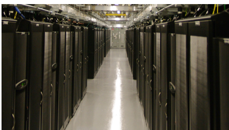
Massachusetts Green High Performance Computing Center (mghpcc.org)
